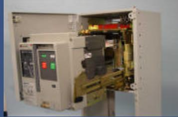
If the breaker switching mechanism itself is in need of replacement, consider installing a form-fit-function replacement using a modern power circuit breaker in the old draw out mechanism. These new circuit breakers can be mounted into a variety of manufacturer's draw out assemblies. This provides a new warranty and because the breaker is of current design, more easily obtained and less expensive spare parts.
