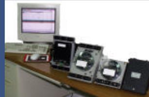
If you have a spot network, you will have network protectors. Old network protectors can be rebuilt with new switching elements and new network protector relays. These new relays substantially reduce the internal wiring, reducing the points of failure, while at the same time providing new diagnostics and protective settings to insure better operation of your spot network.
